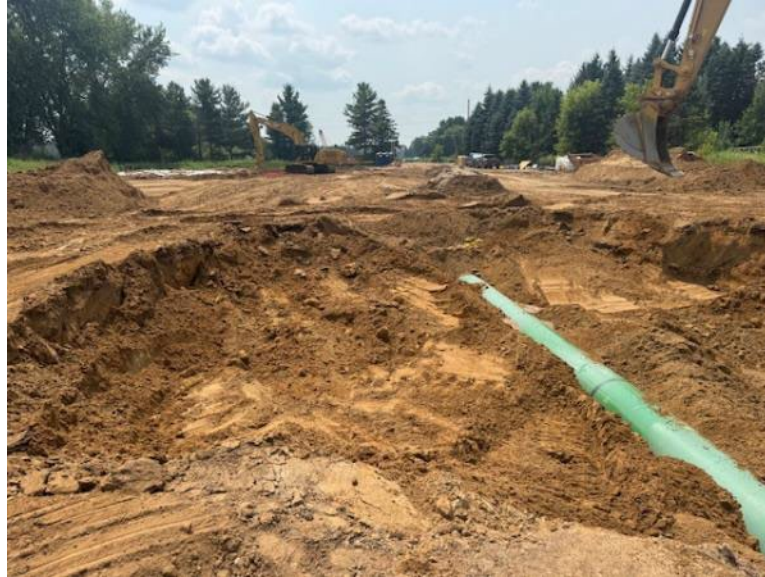
Facing west near MP 3.3, backfill commenced
