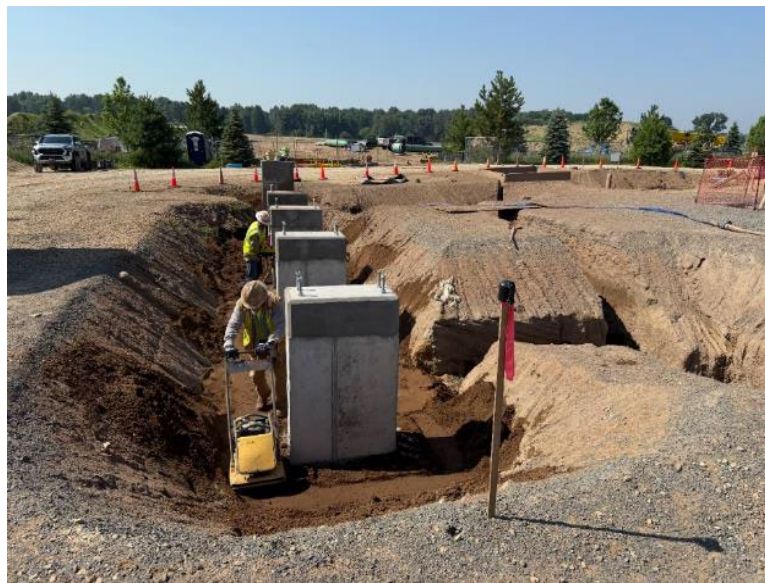
Facing south near MP 0.01, Otis compacting soil around concrete piers
