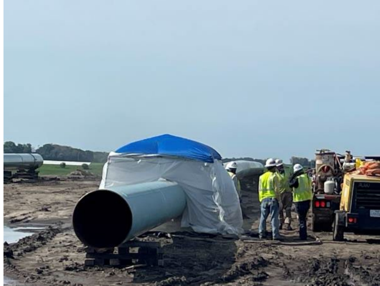
Facing south at MP 33.17, K&K sandblasting and coating mainline pipe south of 154th Street/County Road 80
