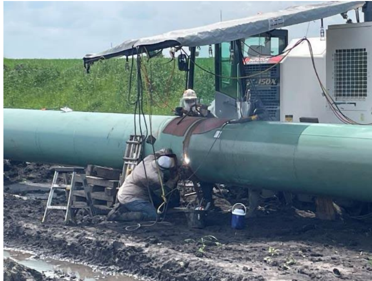
Facing northwest at MP 32.35, K&K welding mainline pipe
