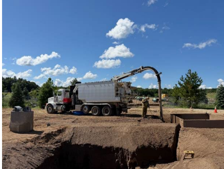
Facing south near MP 0.02, Otis continues hydro vacuum in Hugo compressor station
