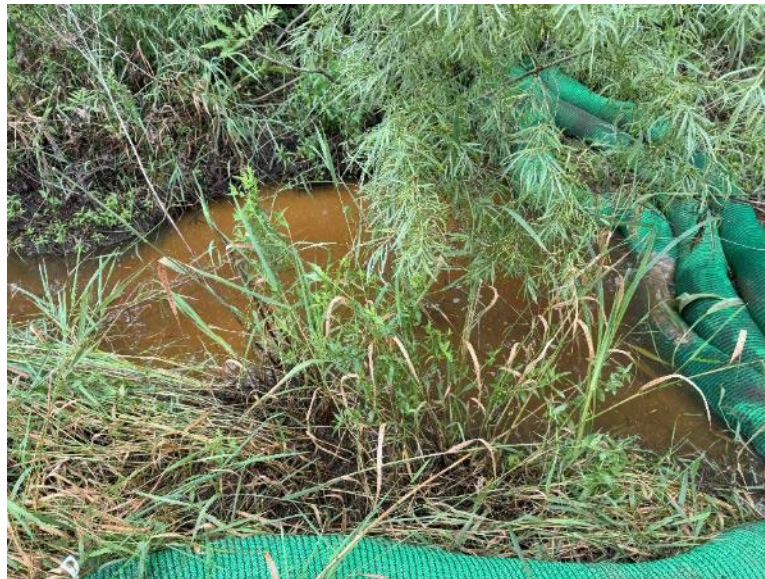
Facing south near MP 2.67, southern terminus of IR drilling fluids contained with silt sock 110 feet from start of release
