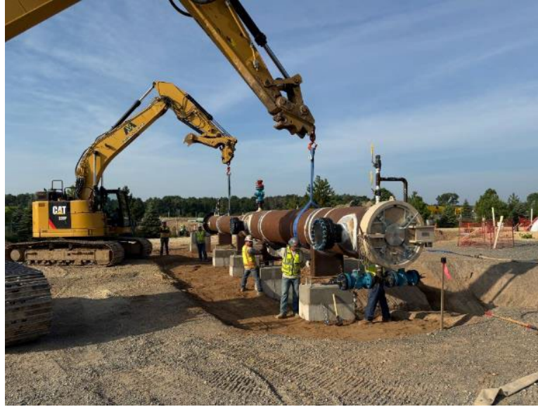
Facing south near MP 0.02, Otis installing the launcher in Hugo compressor station
