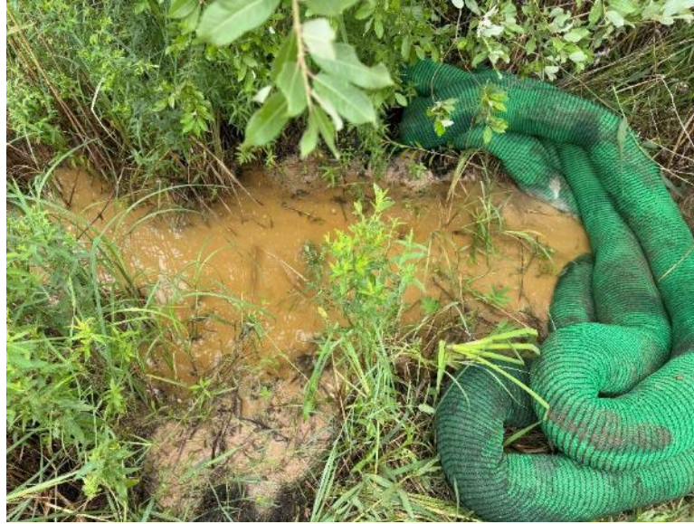
Facing east near MP 2.66, start of IR contained with silt sock
