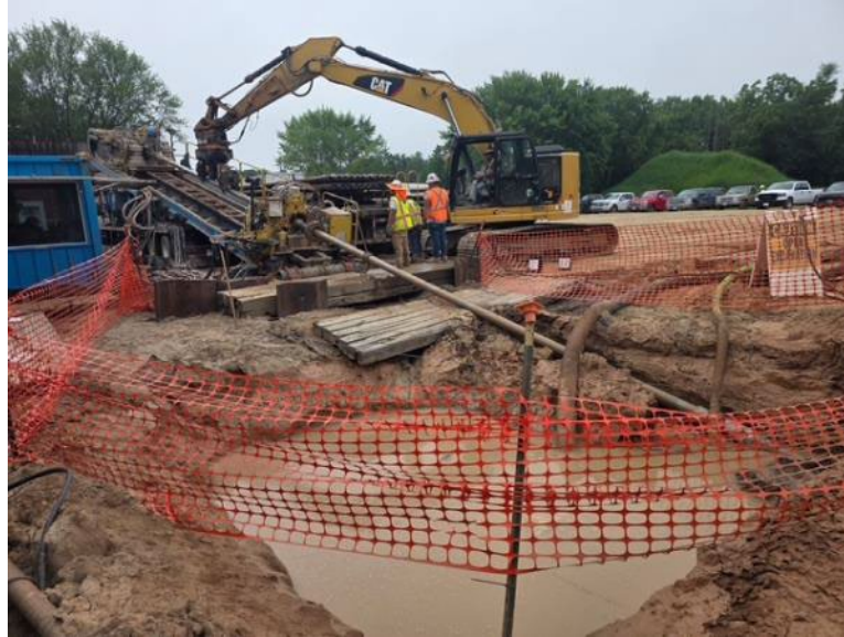
HDD P4-5 continued the pilot pass
