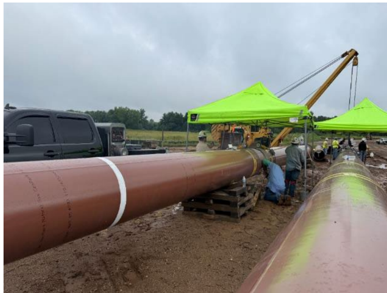
Facing north near MP 0.15, Otis continues welding bore pipe
