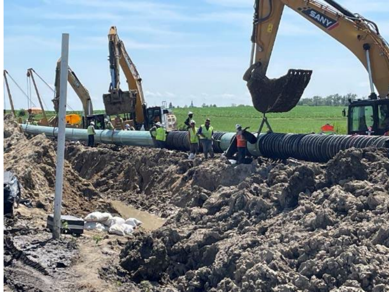
Facing southwest at MP 34.0, K&K lowering-in mainline pipe
