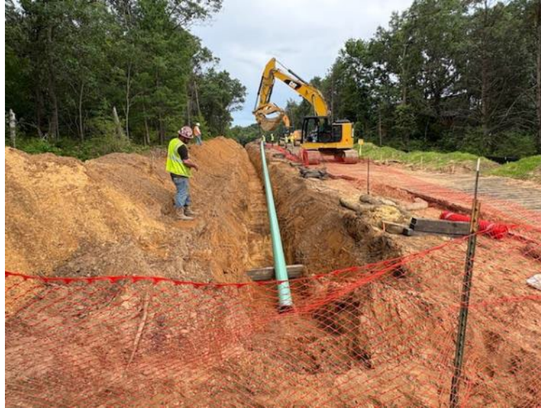
Facing east near MP 2.25, contractor lowering-in pipe
