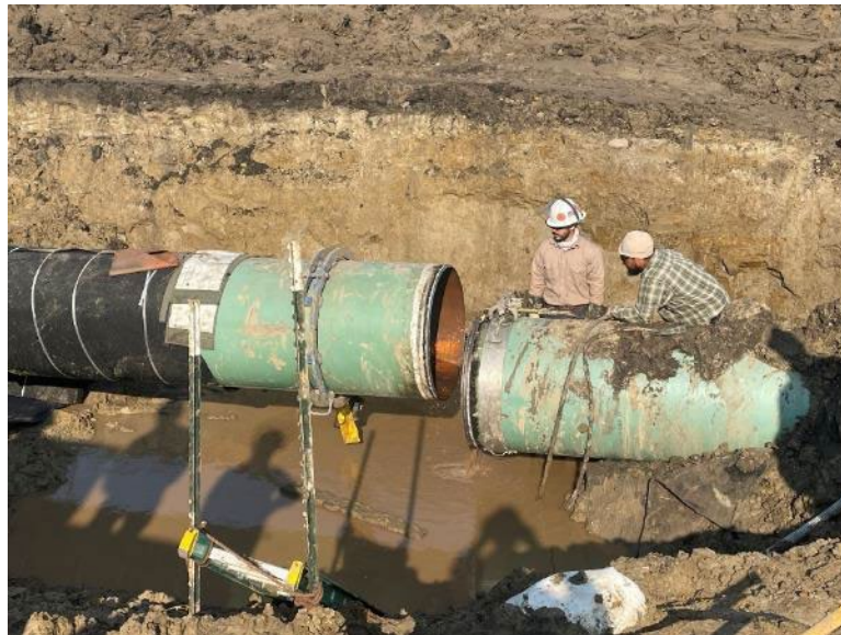
Facing west at MP 34.11, K&K is completing mainline tie-in south of 165th Street
