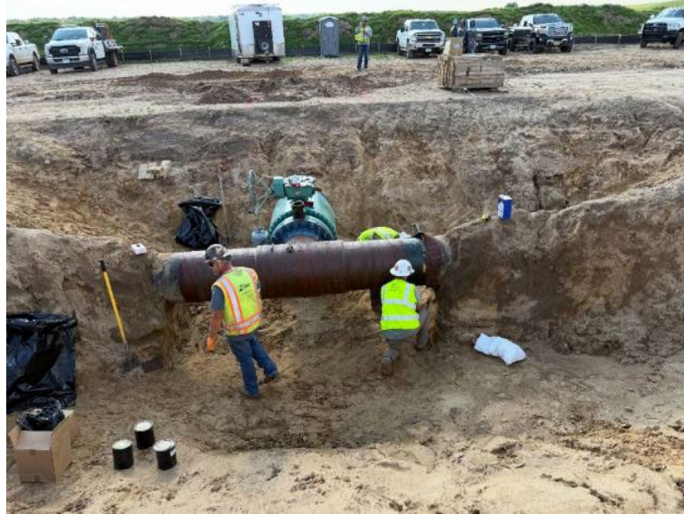
Facing east near MP 1.9, Otis applying wax wrap after completion of the split tee
