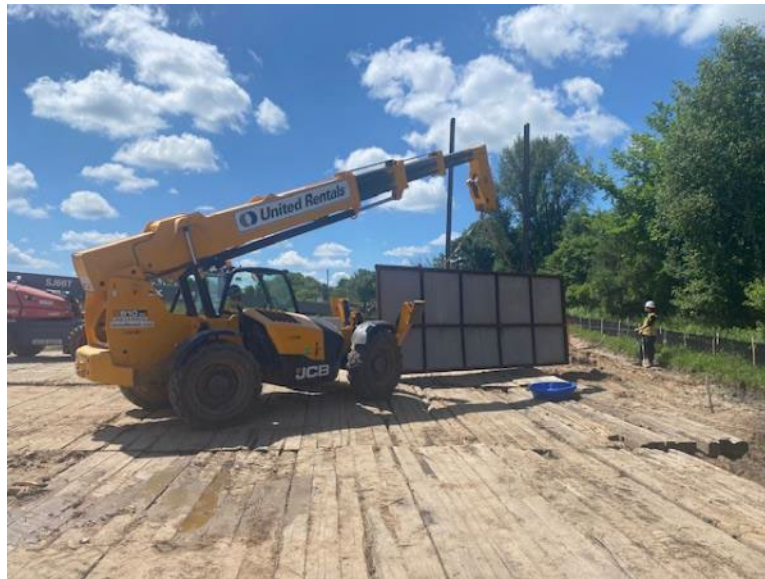
Facing west at HDD P4-2 exit, sound wall installation in progress
