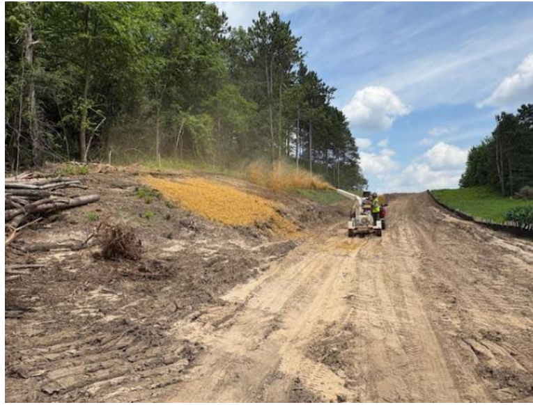
Facing east near MP 3.1, contractor seeding and mulching hillside
