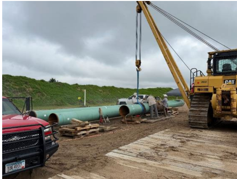
Facing west near MP 1.7, Otis continues stringing line pipe
