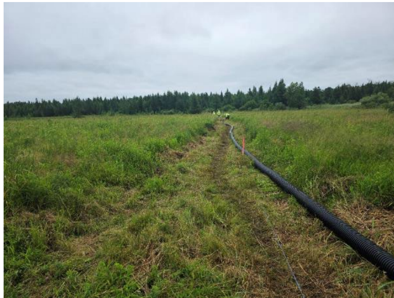
Facing east at MP 2.7, corrugated suction line for the IR response; each connection taped and wrapped with plastic
