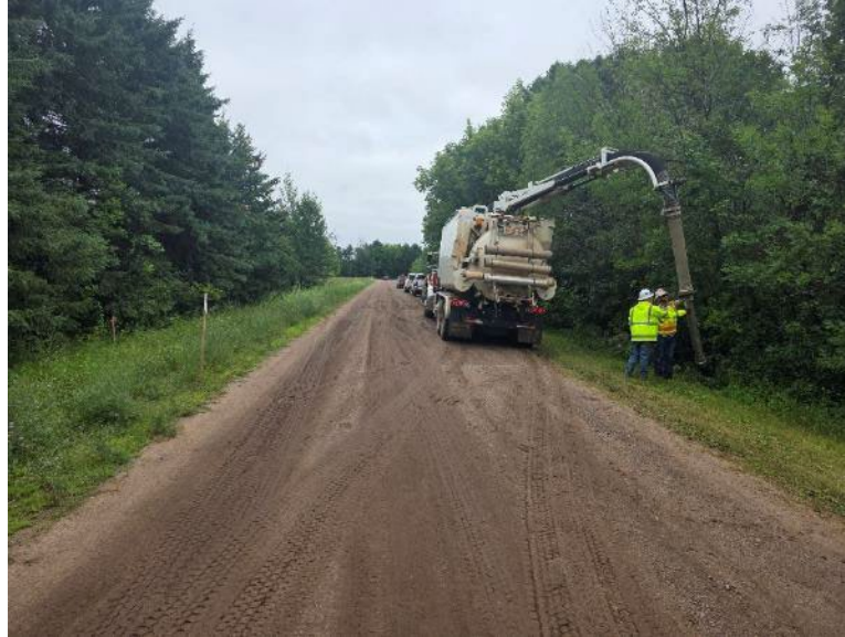
Facing north on 180th North and Imperial Avenue, hydro-vacuum on site for IR response
