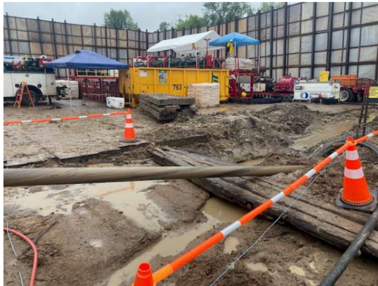
HDD P4-2 completed the pilot pass
